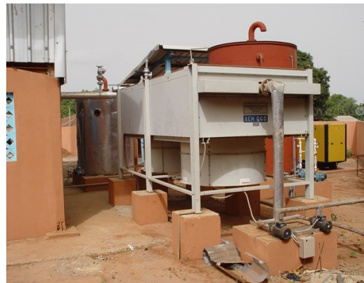
Figure 22: condensador SAFIM
