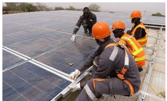
Figure 1 Installation de modules photovoltaïques
