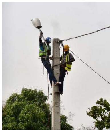
Figure 2 Installation de l'éclairage public
